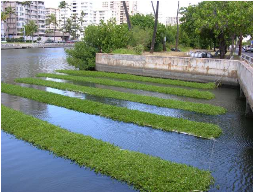
FPP system using salt tolerant Hawaii native plant akulikuli ( Sesuvium portulacastrum L.) clears up runoff polluted Ala Wai Canal in Hawaii.
